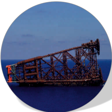
Boyancy tanks Sabratha Construction boyancy tanks Sabratha platform to 27000 t. performed at the Shipyard of Tortoli-Arbatax (OG) in 2003.
