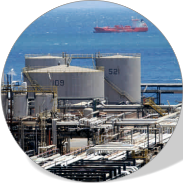
Extraordinary maintenance SARAS Executed in 2009 for extraordinary maintenance of the SARAS S.p.A., petrochemical refinery in Sarroch (CA)
