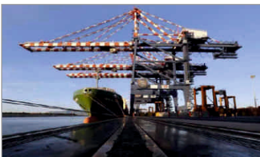
Gioia Tauro harbor cranes | 1994
